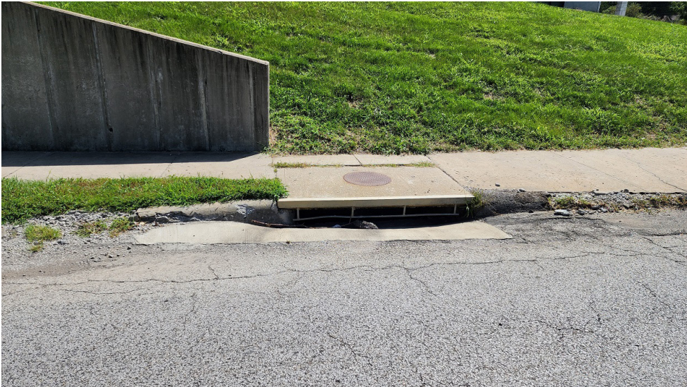
The 59th Street and Raytown Road Stormwater Improvement Project will remove the existing deteriorated stormwater system and replace it with a new concrete pipe system. Some curbing, sidewalks, and ADA ramps will also be replaced. The streets will receive a 2" mill & asphalt overlay at the end of the project. Design of this stormwater project is ongoing, and the easement acquisitions are in progress.
